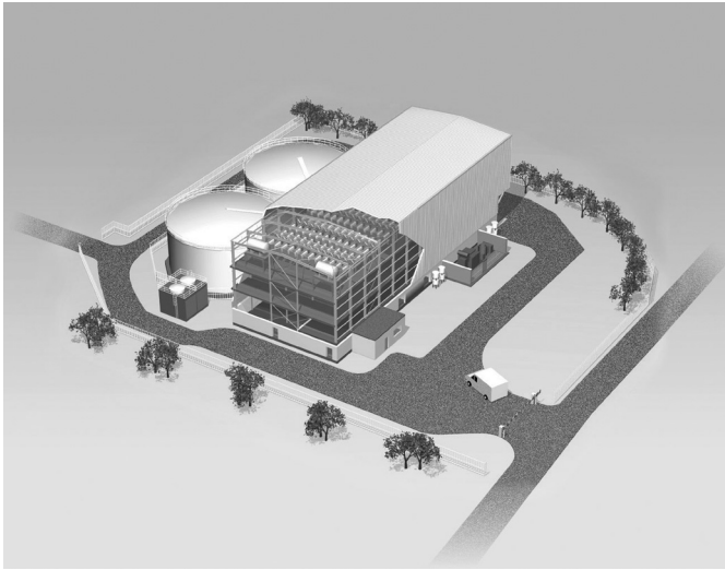
Figure 1.18 Picture of the 100-MWh electrical energy storage facility being installed in Cambridgeshire, England. The storage tanks for the electrolyte solutions ('fuel') can be clearly seen. (Reproduced by kind permission of Regenesys Technology Ltd.)
